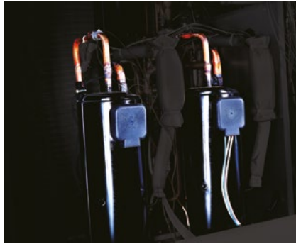
Multiple large-capacity all Inverter compressors (from 14 HP).
