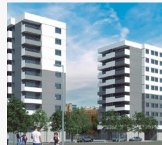
Flumen Plus. Residential passive house building. Zaragoza, Spain. PACi.
