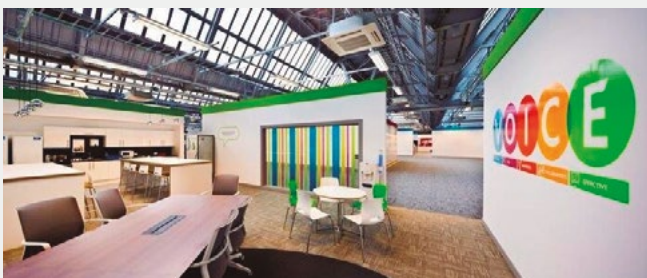
CAPITA call centre. UK. 11 ECO G 3-Pipe units. Over 150 indoor units in meeting rooms and open-plan areas. Intelligent touch screen controller, the CZ-256ESMC2.
