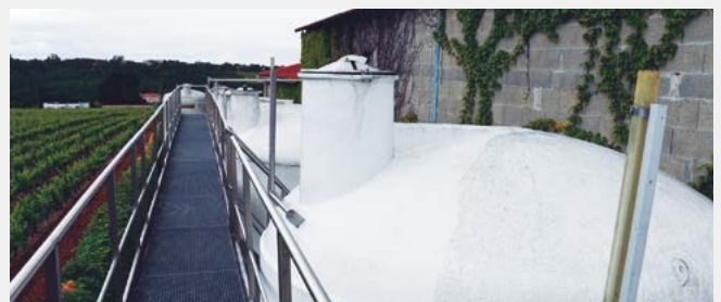
French winery Gennevilliers, France. ECO G 3-Pipe units. One of the best solution utilized our ECO G solution for wine production process.
